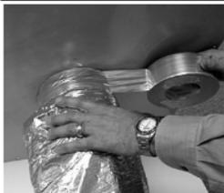
Pull insulation and vapor barrier over connection and secure with 2 wraps of tape labeled as either UL-181A-P or UL-181B-FX or with approved clamp.
