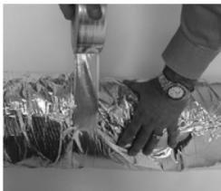
Secure butt joint with 2 wraps of tape labeled as either UL-181A-P or UL-181B-FX.
