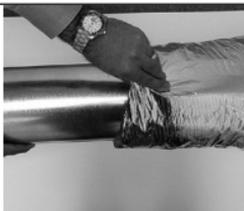
Pull insulation and vapor barrier over starter cap and onto pipe.
