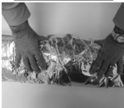
Butt insulation and vapor barriers together.
