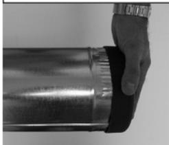
Place plastic starter cap over crimped end of metal pipe section.
